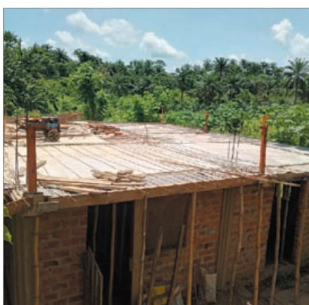
The most difficult and expensive part of the project - laying of the slab for the second floor
