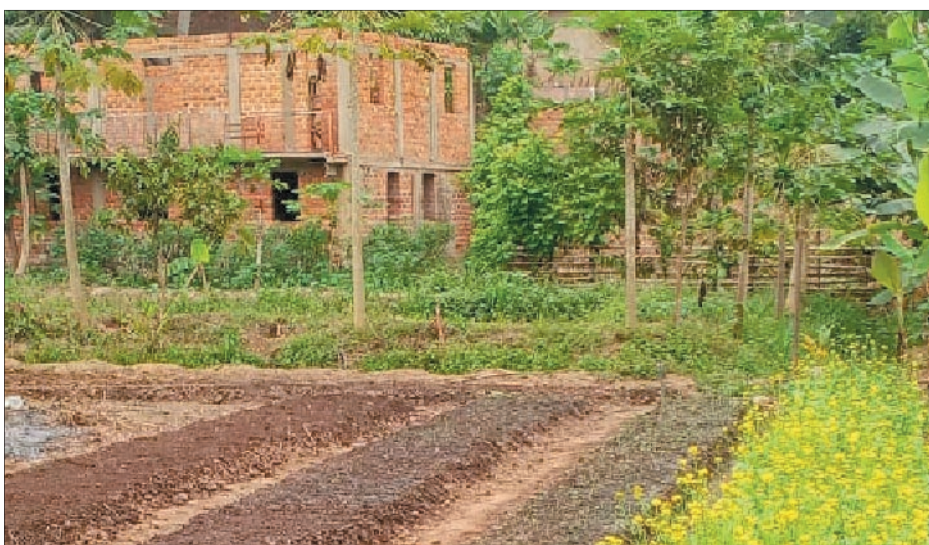
Walls of the second floor are done and ready for the roof
