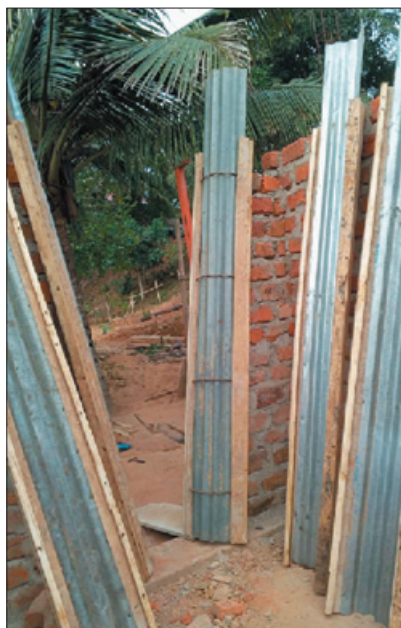
Metal sheets for the columns of the corners are prepared
