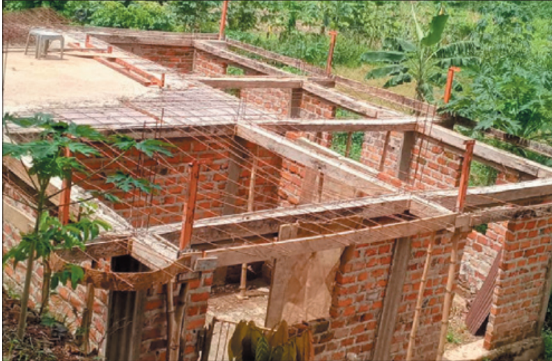
The first part of the slab for the second floor has been laid
