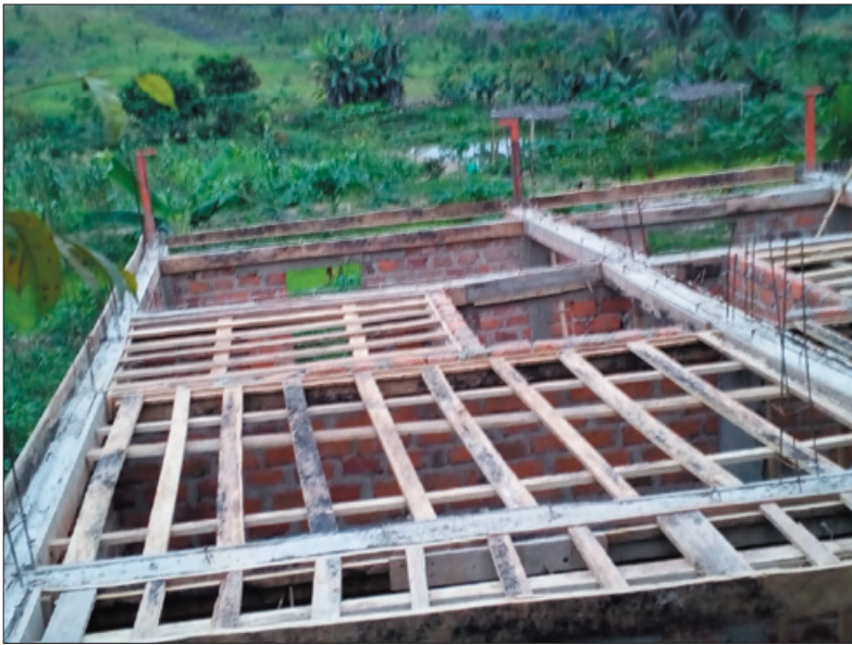
Top - Wooden construction for the 2nd floor
