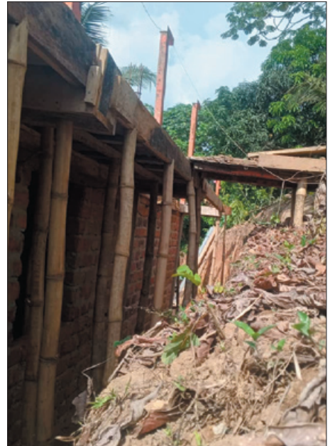
Joseph chopped bamboo to support a structure to hold the slab in its place till the concrete dries up
