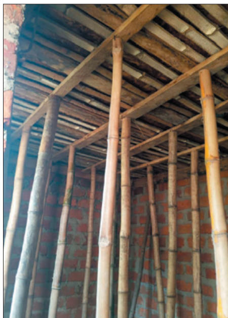
Joseph chopped bamboo to support a structure to hold the slab in its place till the concrete dries up
