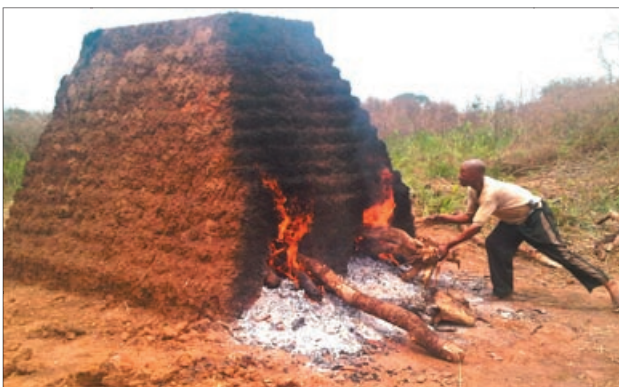
9. Kiln made from bricks on construction site
