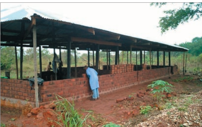
10. Our manager Jean oversees construction
