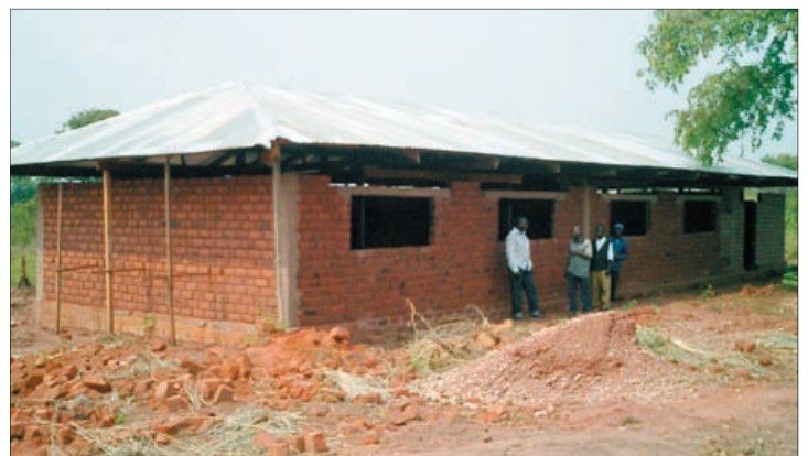
11. Prof. Mpona with foremen at the almost finished building
