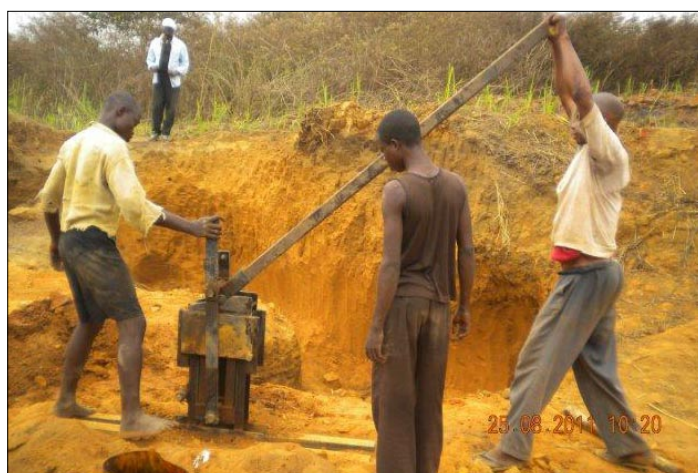
Machine for pressing bricks by hand: clay, a little oil & some elbow grease. After being burned they become very strong
