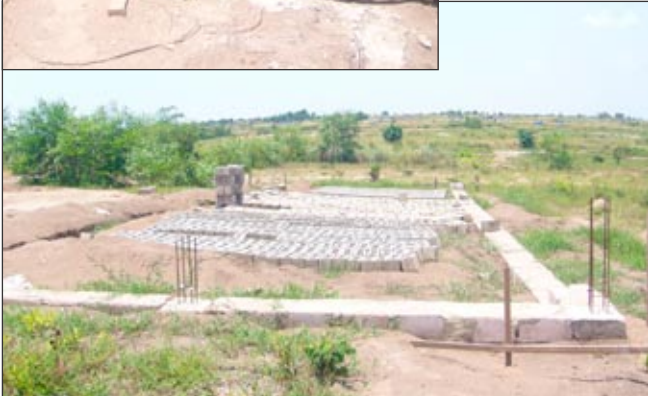
The foundation for the school and bricks for the walls
