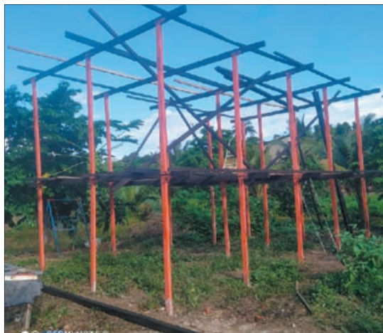
Construction of workshop
