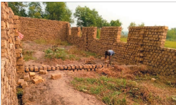
... continued with raising the walls, leaving space for doors & windows with air vents above them, ...
