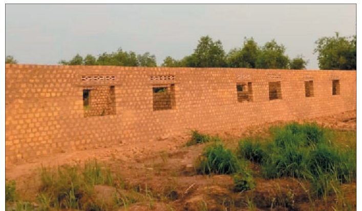
... continued with raising the walls, leaving space for doors & windows with air vents above them, ...
