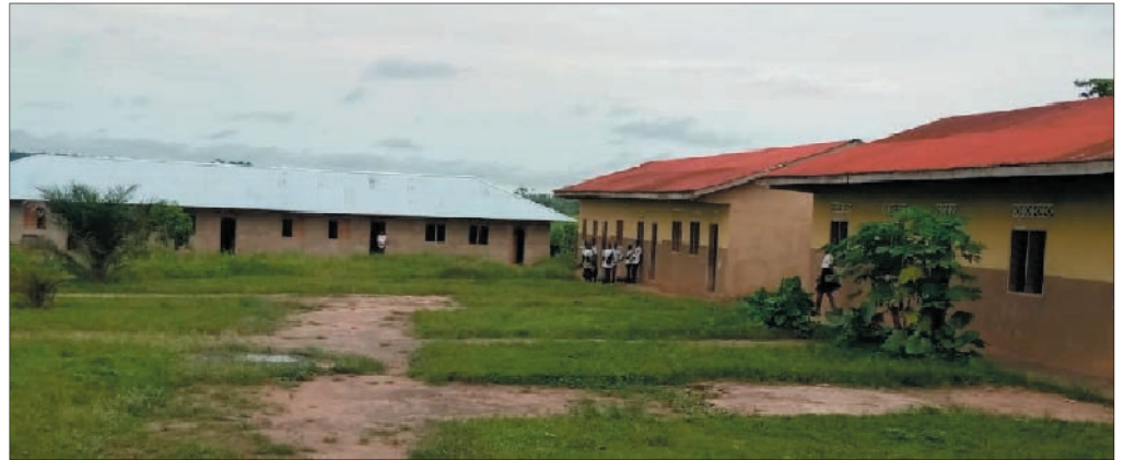
Constructing a new school building with four classrooms (left)
