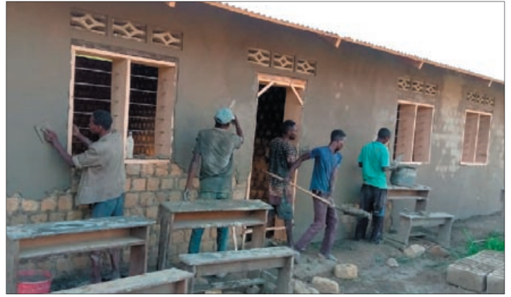
Plastering the walls to protect them against rain
