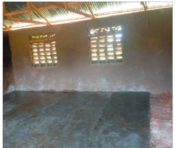
Finishing the inside of the classrooms: Plastering the walls and cementing the floors
