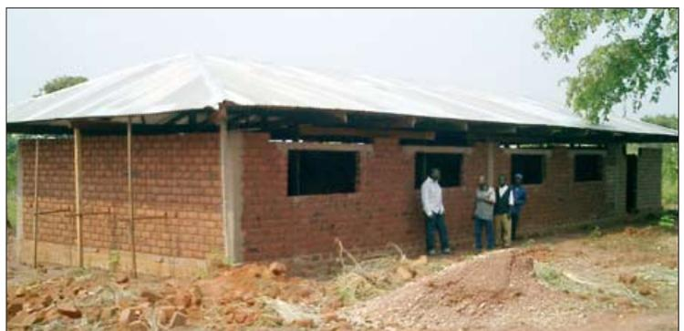
**Left:** First comes the roof to protect the construction from the rain, then the walls go up. **Right:** ... almost finished now!
