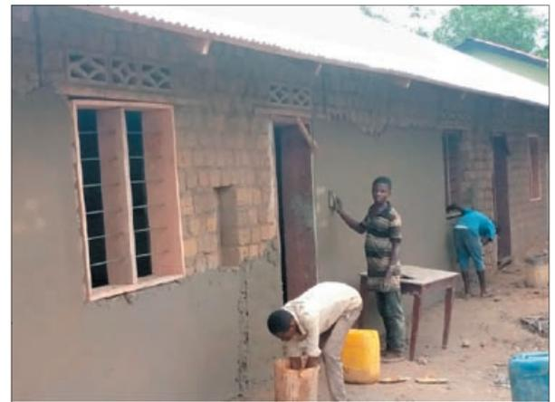
*Plastering the walls for rain protection.*
